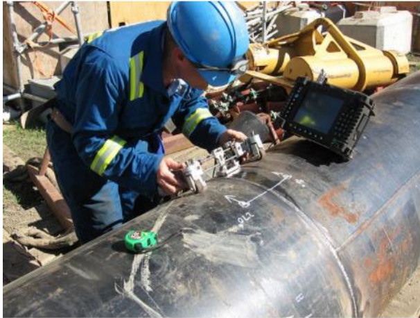
Figure 93. Ultrasonic Testing of a Pipeline
